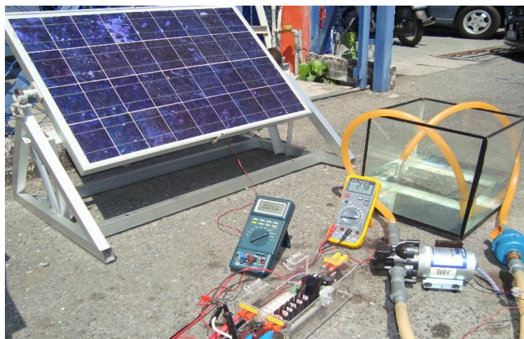
Fig 8: Experiment of DC water pump running with LCB and current multiple circuit
