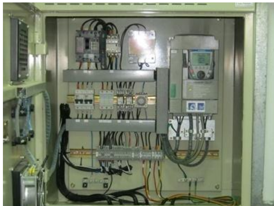
Fig 9: Power circuit
